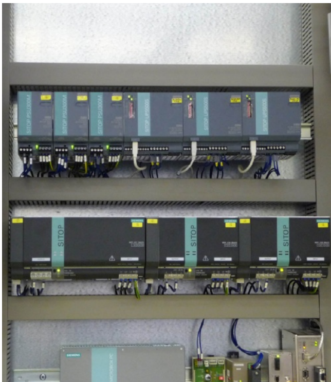
DIN rail mounting of 3 compact SITOP UPS500S basic units together with SITOP modular switched-mode power supplies
